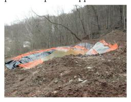
Material must stay in the pit. Overspray of waste or drill mud must not happen.
