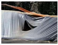
Improperly constructed pits will have stormwater drainage from the site into the pit. Pit failures are evident when part of the pit wall collapses or slumps into the pit, or when the pit or part of the pit has slipped on a fill slope.
