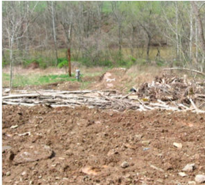
Photograph 6. This was taken looking north from the closed pit. The main and the smaller side log piles are visible, as is the separator for well 731. The drainage ditch to the east of the separator drains the flat that 731 sits on. The Pocatalico River is visible through the trees.
