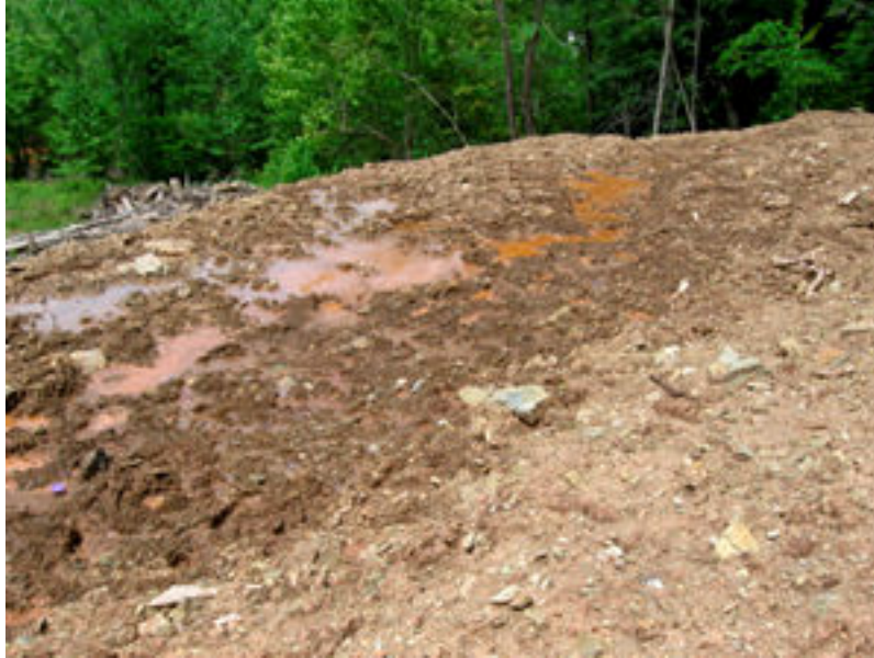
Photograph 5. This is the closed pit, looking toward the northeast corner as in Photograph 4. Standing water is readily apparent. The main drainage point is to the left edge of this photograph. Secondary drainage points are to the east and northeast sides of the closed pit area.
